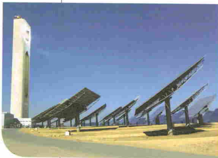
Solar collectors capture energy from the sun at a solar-thermal power station.
