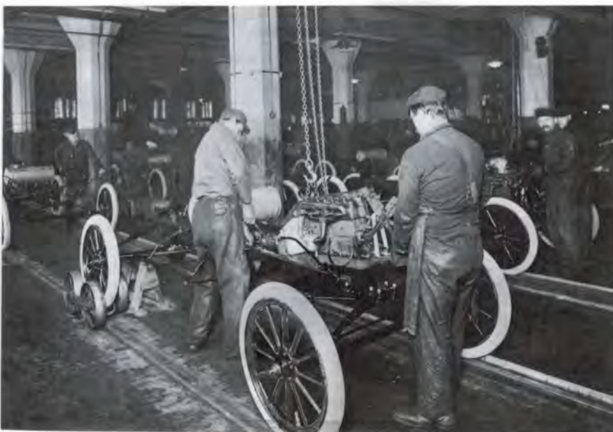
Henry Ford's Model T assembly line
