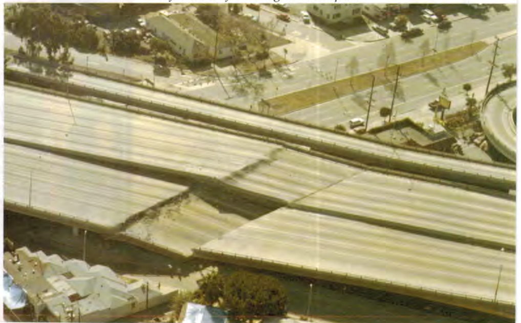
Aftermath of Los Angeles earthquake
