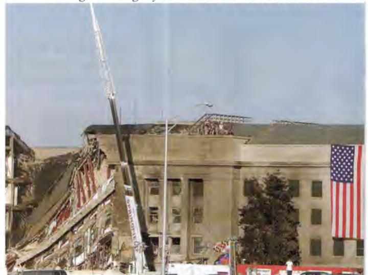
Pentagon damage after the "9-11" terrorist attacks
