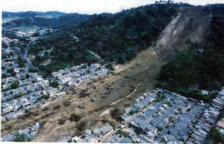
Figure 22 The damage here was caused by a landslide that was triggered by an earthquake.
